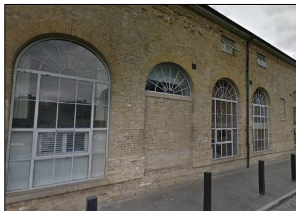
The former Goods Shed has been redeveloped
